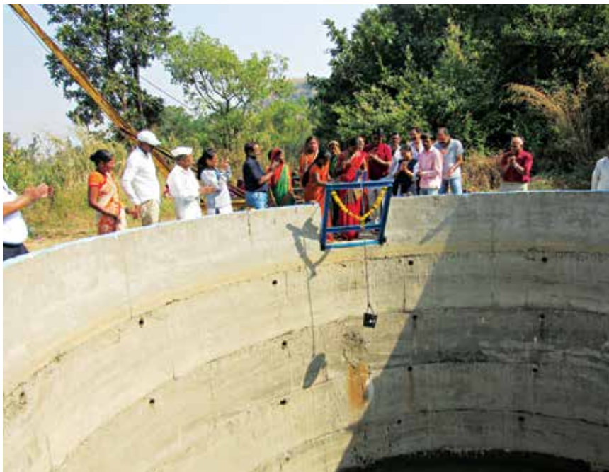
Well construction - Rural development project
